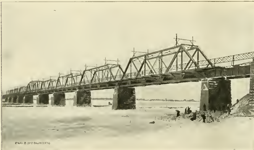
LAURIER BRIDGE ON THE CHATEAUGAY & NORTHERN, NEAR MONTREAL.
